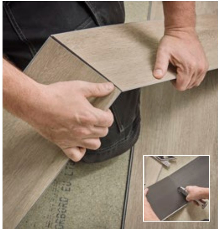
2. Score the plank once and snap it so you have the desired length. Turn the plank over, using a knife fully separate the backing.
