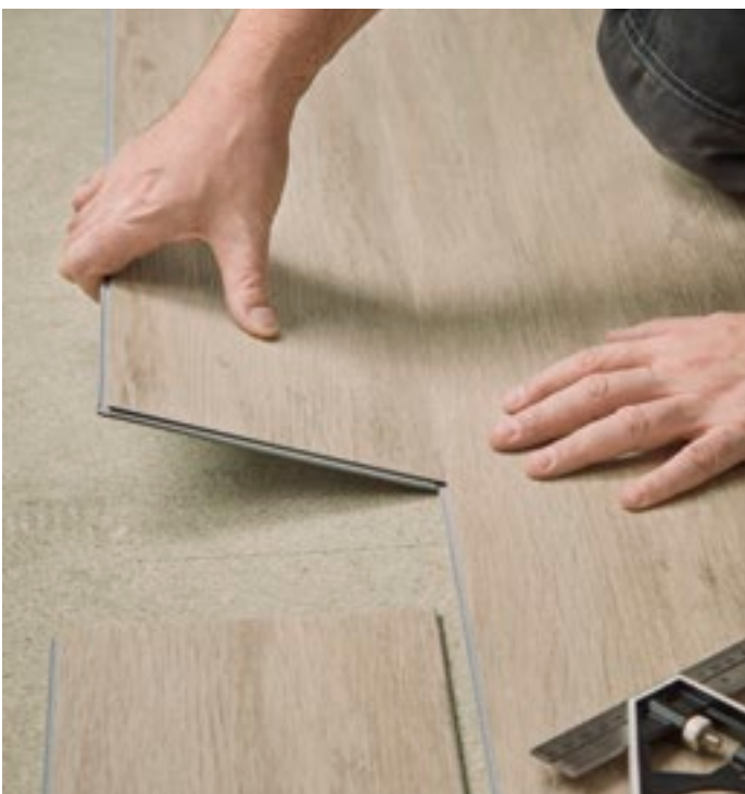
3. No need for adhesive, click and lock the planks into place.
