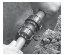
5. Pipe Insertion Insert the pipe fully into the fitting to the point where the stop is felt.
