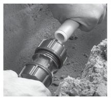
**4. Ready to Use Position** The fitting is pre-assembled and ready to use, however always ensure the nut is fully relaxed and 2 threads are showing before inserting the pipe.
