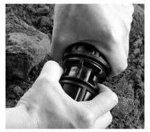
5. Nut Tightening The nut should be tightened by hand and then firmly with a wrench.
