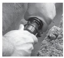
6. Nut Tightening The nut should be tightened by hand and then firmly with a wrench.
