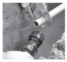
I. Cut the Pipe Square Cut the pipe square. There is no need to prepare the pipe end. Chamfering or lubrication is not required.
