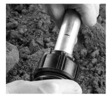
**4. Pipe Insertion** Insert the pipe fully into the fitting up to the witness mark.
