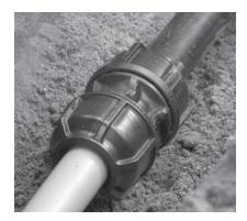
8. Imperial Fully Installed For connections to Imperial PE pipe (BS1972/3284 and IRS 135 Heavy Gauge) steps 5 to 8 are the same as for MDPE connections.
