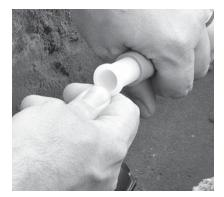
2. Insert Liner in MDPE pipe With MDPE pipe a liner must be used to ensure conformance with WRAS.
